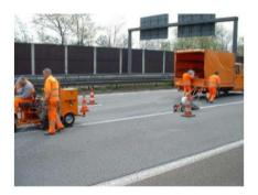
For the application of the Stamark<sup>™</sup> tape the usage of the Manual tape applicator MTA-2 is recommended to assure best results
