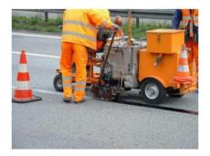
The thickness of the Bitumen layer is related to the surface roughness. Consumption of the Bitumen is strongly depending on the surface roughness. It can be calculated as written in the technical datasheet. Typical values for a 2mm Bitumen thickness are: 42g Bitumen per cm Bitumen layer width and linear meter.
